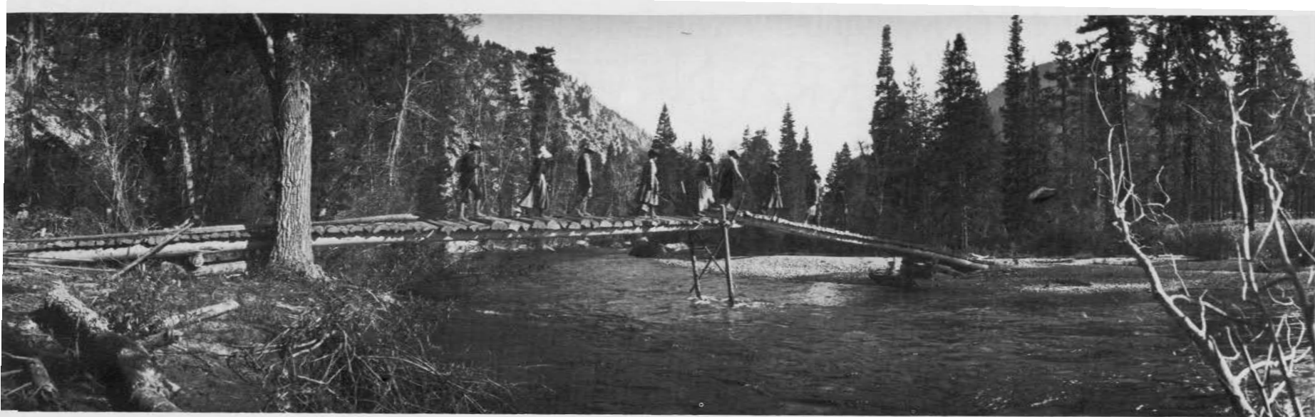
Temporary footbridge at Horse Crossing above Lewis Camp.
